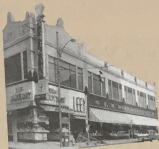
The nationally registered F.W. Woolworth Building, Greensboro, N.C., is the site of the first civil rights lunch counter "sit-in" in 1960.
